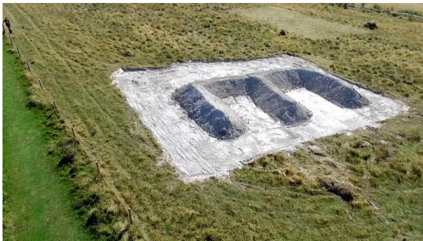
Newly constructed invertebrate bank
